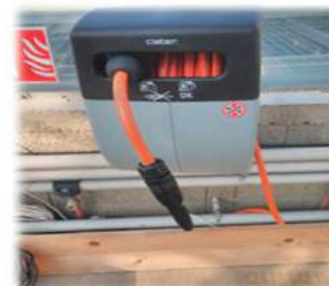
Tuyau de rinçage (bord des bassins)
